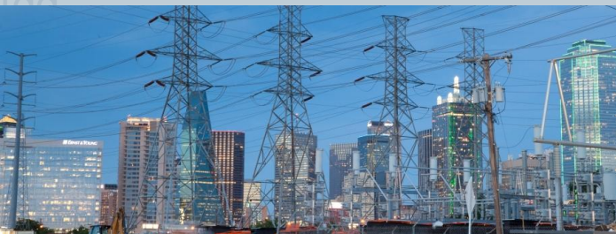
Siemens aims to lower the loss of energy during transmission worldwide to 3% from the current 6,5 - 12%
