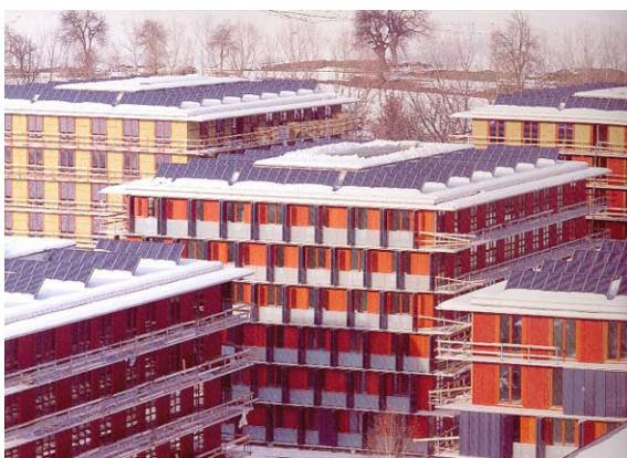
Figure 1. Compact housing form in Hötting West
