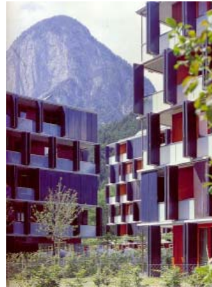
Figure 5 Operable façade in Hötting West
